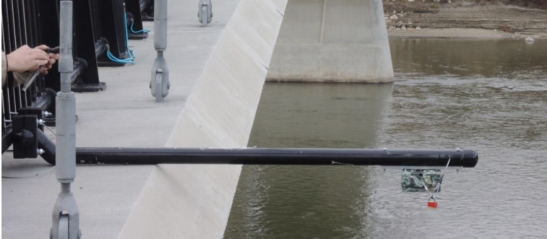
Figure 3-4. Digital image showing the PVC pipe game camera mount on the Fort Edmonton Footbridge. Game camera mount extends ~1.4m from the bridge railing.
