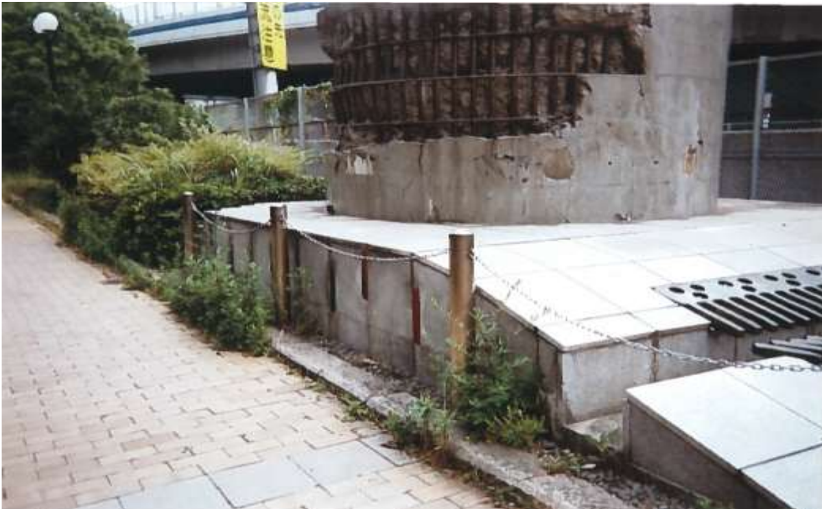
Broken pillar under a highway (Photo taken by Ama)
