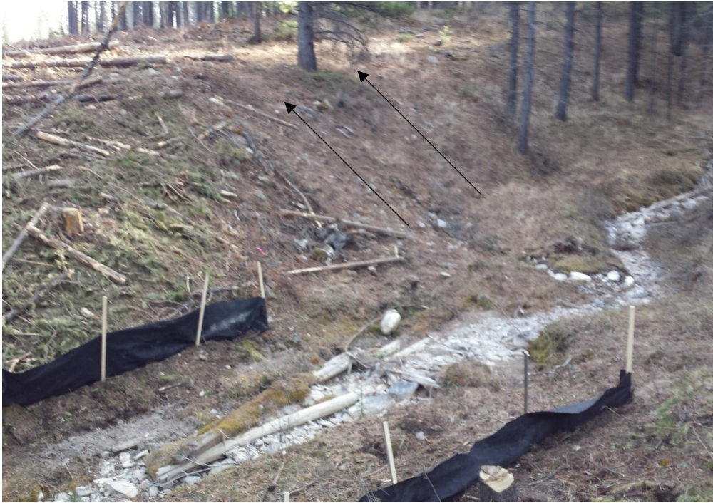
Figure 2-10. Photograph of backhoe cat tracks present on valley banks in McLaren Creek.
