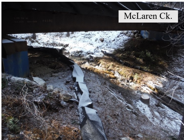
Figure 2-2. Single span two-girder bridge crossings in Star West (9 m, top), Star East (10 m, middle) and McLaren Ck. (15 m, bottom). Bridges were wrapped in geotextile fabric.
