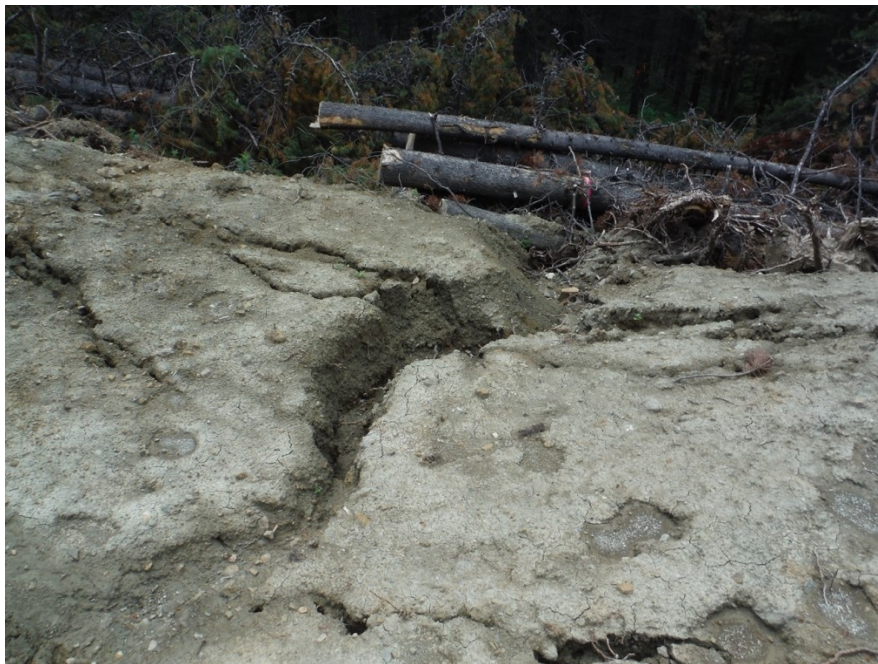
Figure 2-13. Hillslope woody debris retaining sediment-laden runoff from temporary water-bar network.
