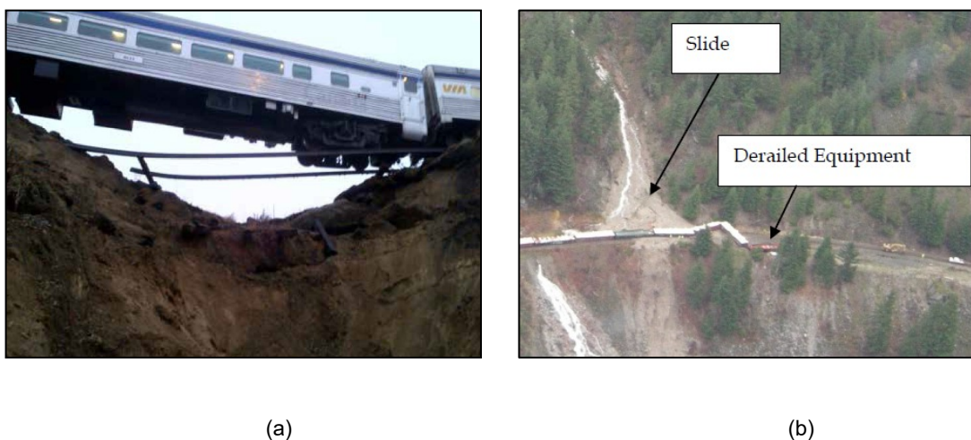
Figure 5-11. Examples of common ground hazards incidents: (a) subgrade washout; and, (b) debris slide on track. (Source: TSB Railway Investigation Reports R13W0124 and R09V0235)
