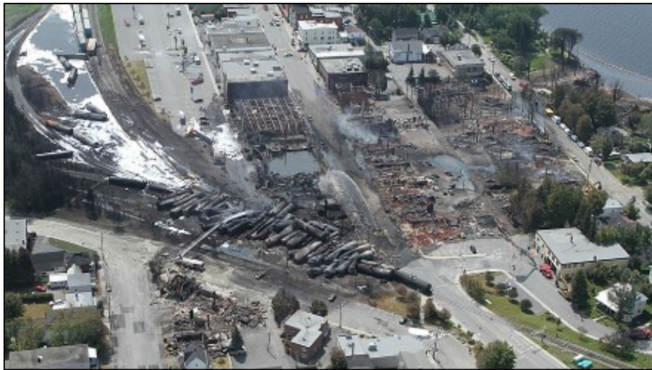
Figure 1-2. Downtown Lac Mégantic after derailment and subsequent explosion.
