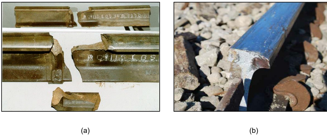
Figure 5-5. Examples of common rail break type failures: (a) failure initiated at weld; and, (b) transverse defects. (Source: TSB Railway Investigation Reports R99H0010 and R11C0118)
