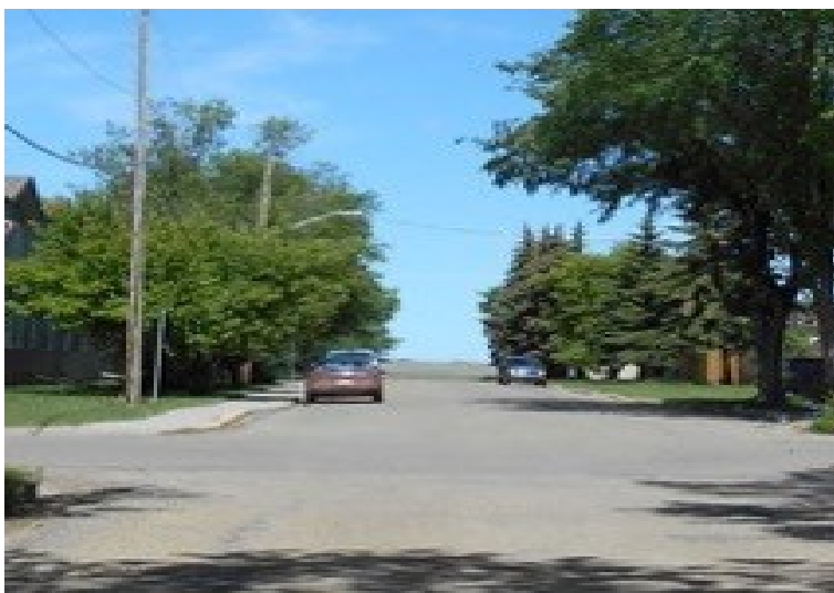
Figure 18. No road signs
