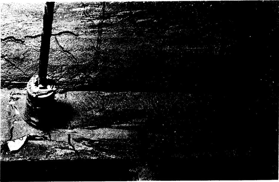
Fig. 8.12 Inclined Cracks in Wall
