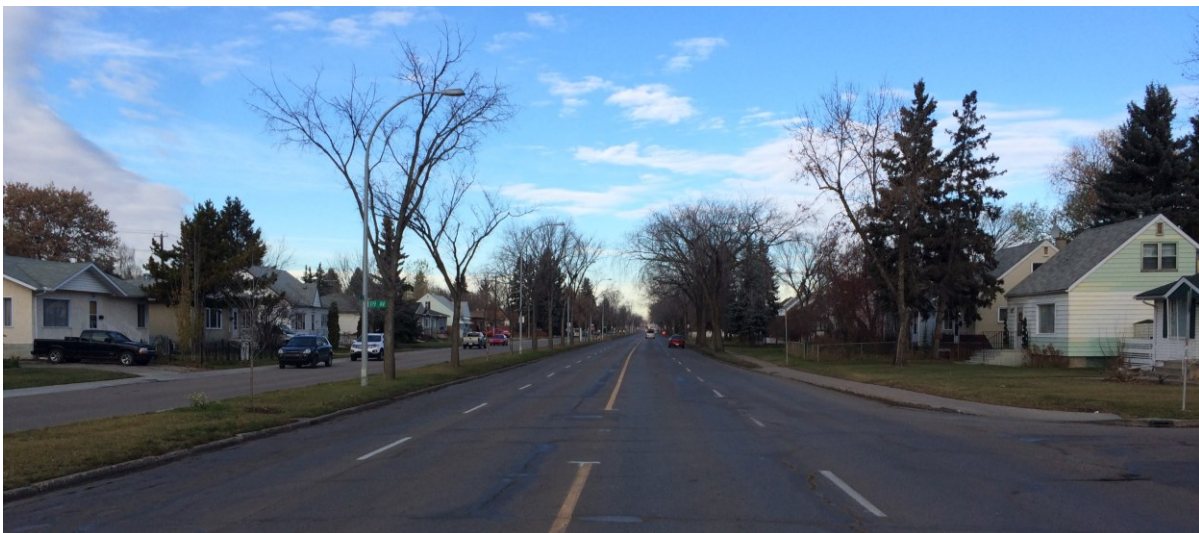
127 Street at 119 Avenue: undivided arterial with single service road
