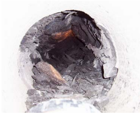
(c) Long-term development associated with strength degradation of bedding.
