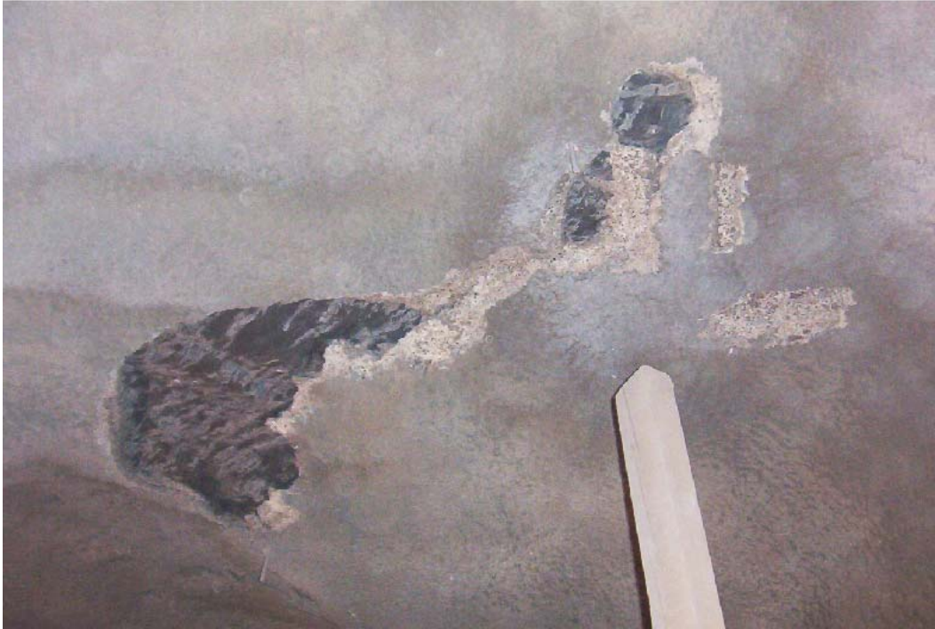
Figure 1.8: Cracking and debonding of shotcrete in the roof of the Starter Niche at Mont Terri more than a week after installation. This demonstrates the time-dependent behaviour of tunnels in Opalinus Clay.
