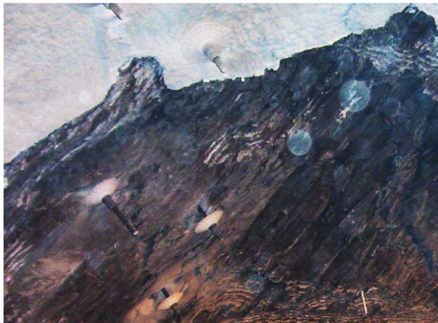
(b) Anchored support was required for upper left corner of excavation.
