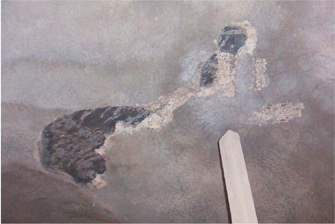
Figure D.4: Cracking and debonding of shotcrete in roof of Starter niche. Face of excavation is approximately 25 m beyond this location.
