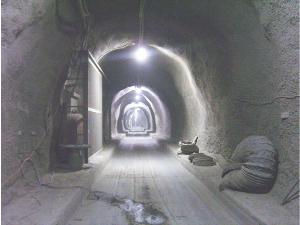
Figure D.7: Looking towards the northwest along the Security Gallery.
