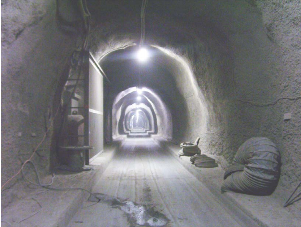
Figure 1.6: Looking towards the northwest along the Security Gallery.
