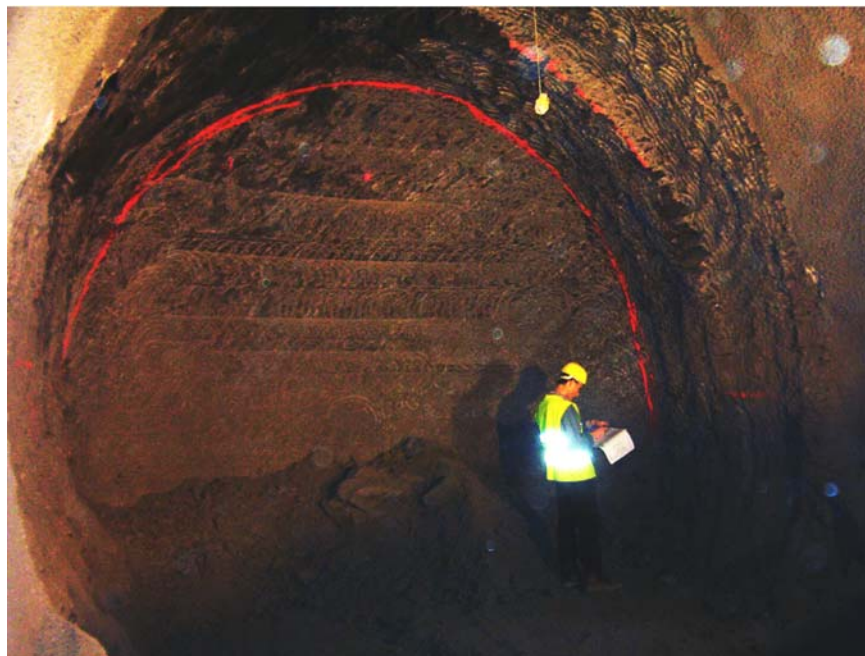
(b) Some structurally controlled instability in upper left corner, but none in the excavation face.
