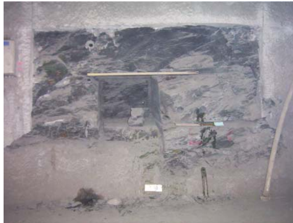
(b) Shotcrete was cut out in OP niche for investigation. A large block sample was removed from centre area of picture.
