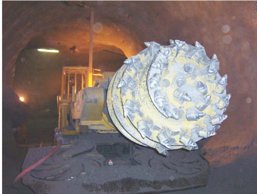
(a) A roadheader was used for mechanized excavation.
