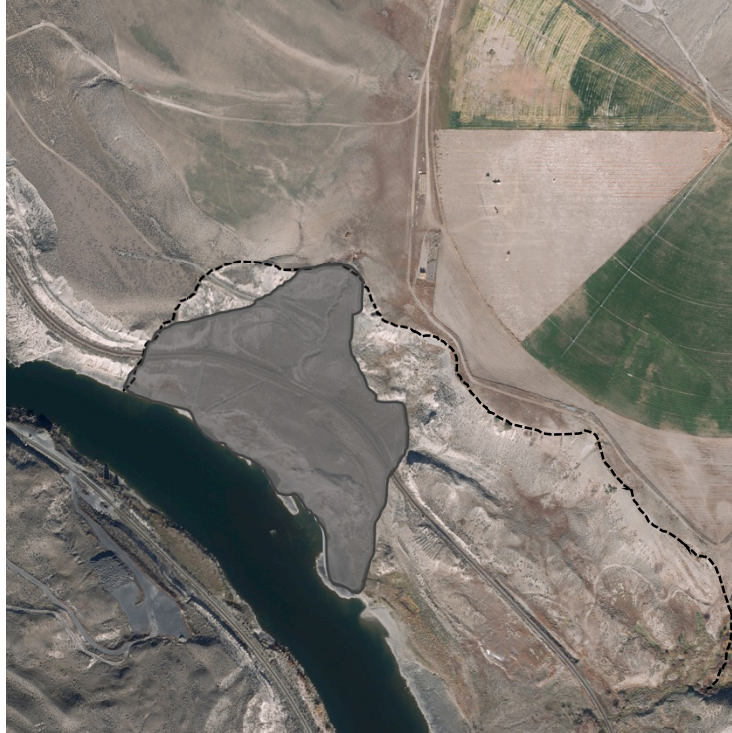
Figure 3.6: 2015 aerial photo of the Goddard landslide on the east bank of the Thompson River (courtesy of CN rail); shaded area corresponds to the limits of the 1982 reactivation (as per Eshraghian et al. (2007)), dashed line delineates broader extents of an older, possibly ancient landslide feature.
