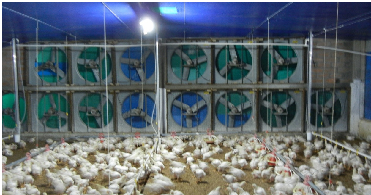
Figure 4.3. Tunnel-ventilated house with foggers.
