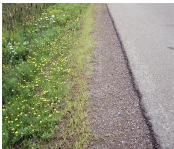
Figure 6.5. Photograph E, unsafe shoulders for walking and biking
