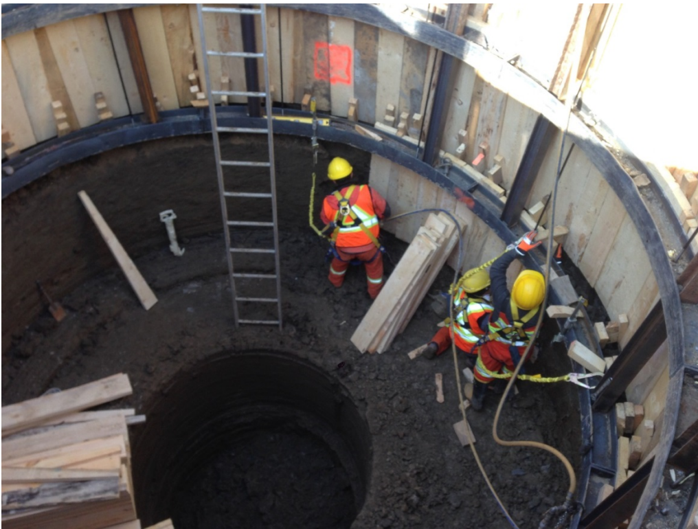
Figure 11: Rib by rib drill rig assisted excavation of a working shaft
